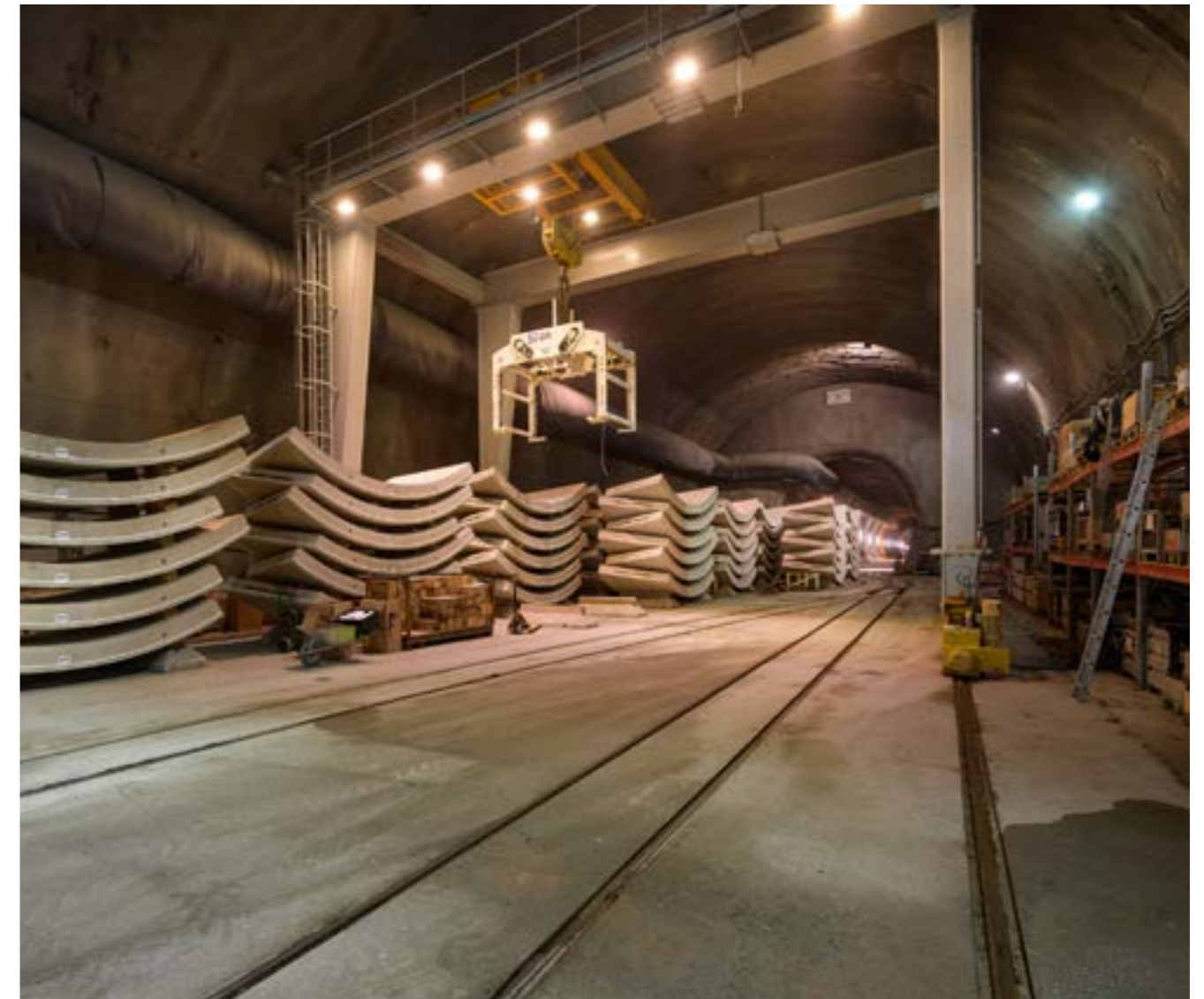
The emergency stop in the Fröschnitzgraben area is currently under construction
