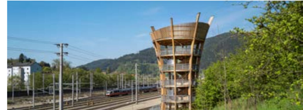
A splendid overview of the construction site can be observed from the information tower in Müzzuschlag.
