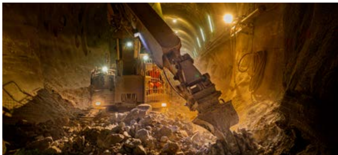
A major part of the tunnel was created via excavation and blasting.
