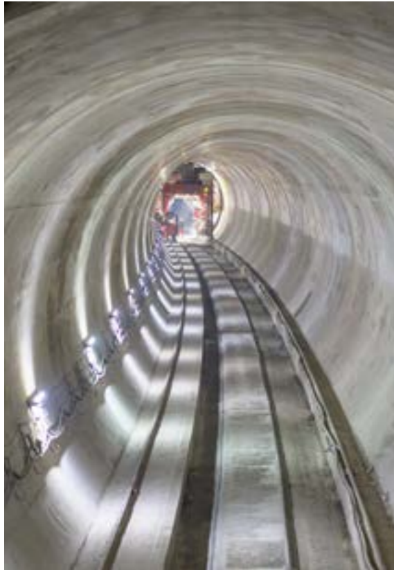
Parts of the tunnel inner lining have already been built
