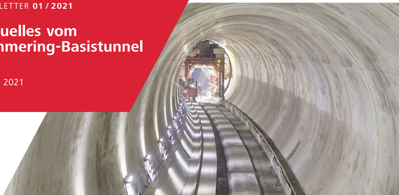
Innenschale in Gloggnitz
